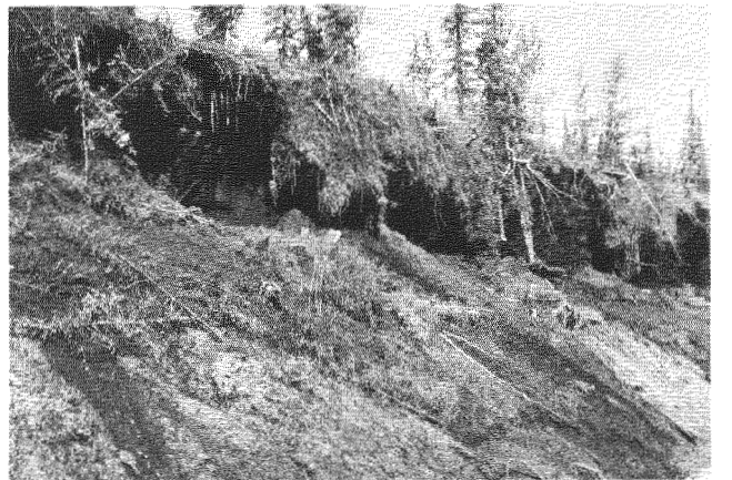
FIGURE 13 Massive ice under overhang, 32.6 km, 11 August 1970.
