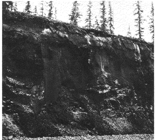
FIGURE 9 Frozen vertical backslope, 32.6 km, 23 April 1970.
