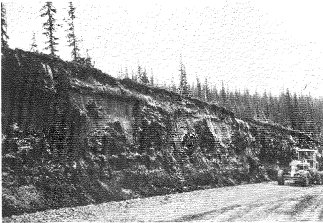
FIGURE 10 Frozen vertical backslope, 32.6 km, 23 April 1970.
