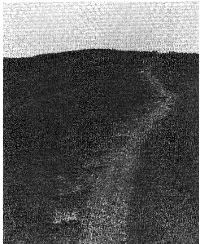
FIGURE 2 Effective water bar constructions on fireline in ice-rich permafrost.
