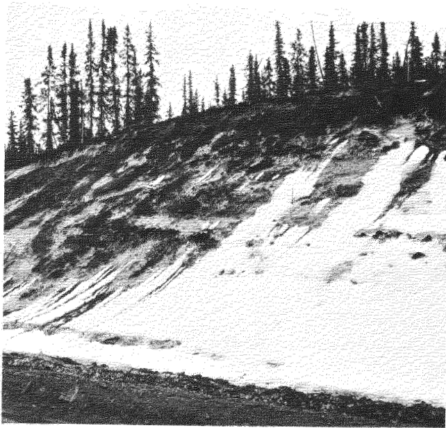
FIGURE 3 Frozen 1:1 backslope, 31.6 km, 23 April 1970.
