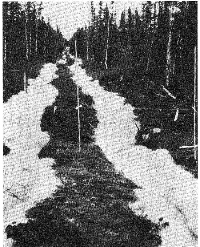
FIGURE 4 Same trail identified in Figure 3 after application of seed and fertilizer covered by excelsior mulch.
