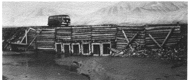
FIG. 2. Roads contain large culverts to handle flash floods.
