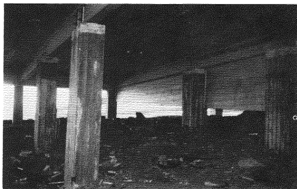
FIG. 7. View of the underside of the building shown in Figure 6.
