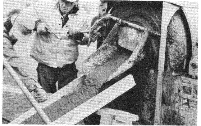
FIG. 4. The sand slurry left the mixer the consistency of wet concrete.
