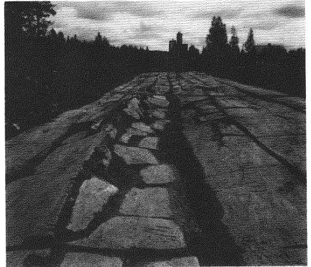
Fig. 6. A photo of a decovered damaged layer of plastic foam, where the separate boards have slid apart, so that openings have arisen.
