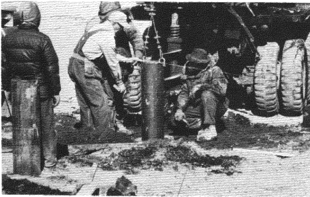
FIG. 3. Alignment was checked before the slurry backfill was added.
