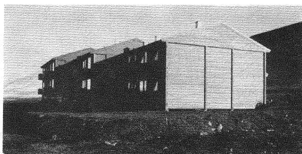
FIG. 6. Apartment supported on a concrete post and pad foundation.
