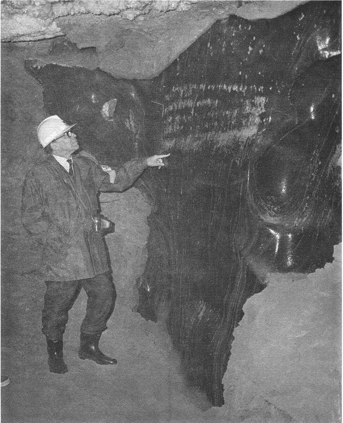
Fig. 1. Foliated ice wedge exposed in permafrost in experimental tunnel near Fox, Alaska excavated by U.S. Army Cold Regions Research and Engineering Laboratory. Temperature in tunnel 0.5^{\circ}\text{C} . (Photograph by C. J. Romberg, 1973)
