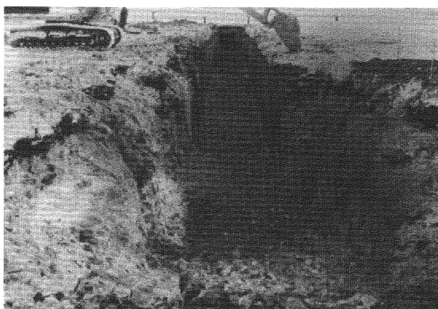
Figure 7 Rocsaw cut and blasted section.
