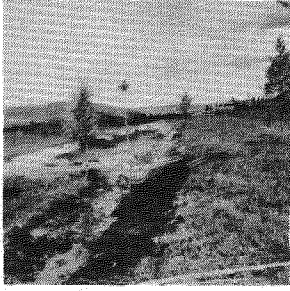
FIGURE 3 Wide, shallow, large-sectioned drainage ditch.
