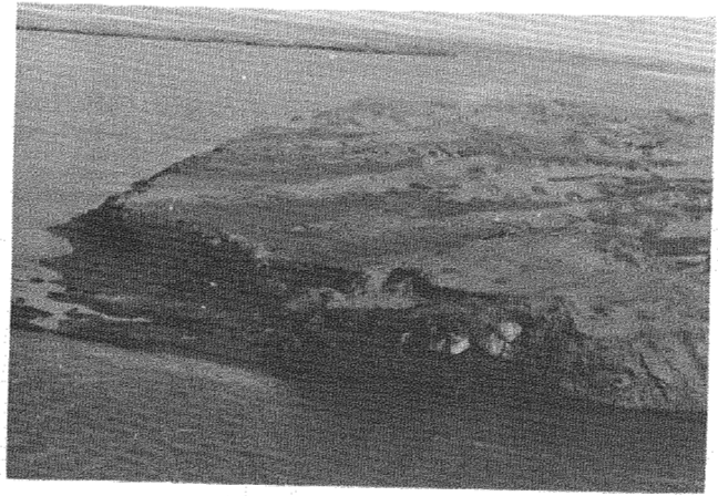
FIGURE 16 Photograph of erosion at the south end of the island at site 6.
