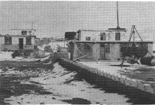
FIGURE 12 Water-supply system with heat-preserving pipes on ground and outside cistern.
