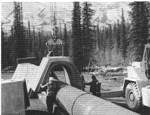
FIGURE 13 Construction of above-grade, concrete restrained mode at Quill Creek Test Facility.
