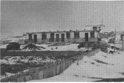
FIGURE 10 High-filled, ventilated foundation test structure.
