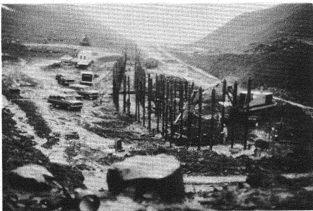
FIGURE 7 South Repair Area (Looking South)
