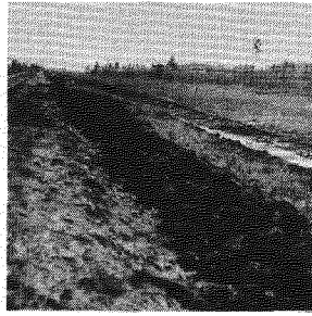
FIGURE 4 Thermal-insulating revetment road without soil covering.
