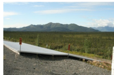
Figure 7. Snow/Sun shed on the west side of the Alaska Highway.
