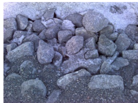
Figure 10. West slope of the ACE uncovered contaminated with gravels by snow removal in March 2011.
