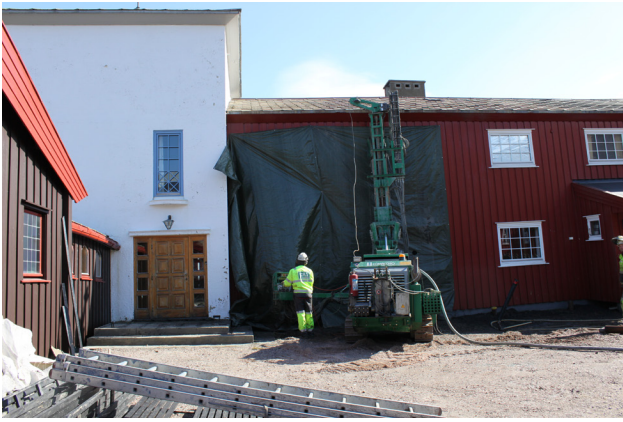
Figure 4. Sysselemannsgården during reconstruction of foundation.
