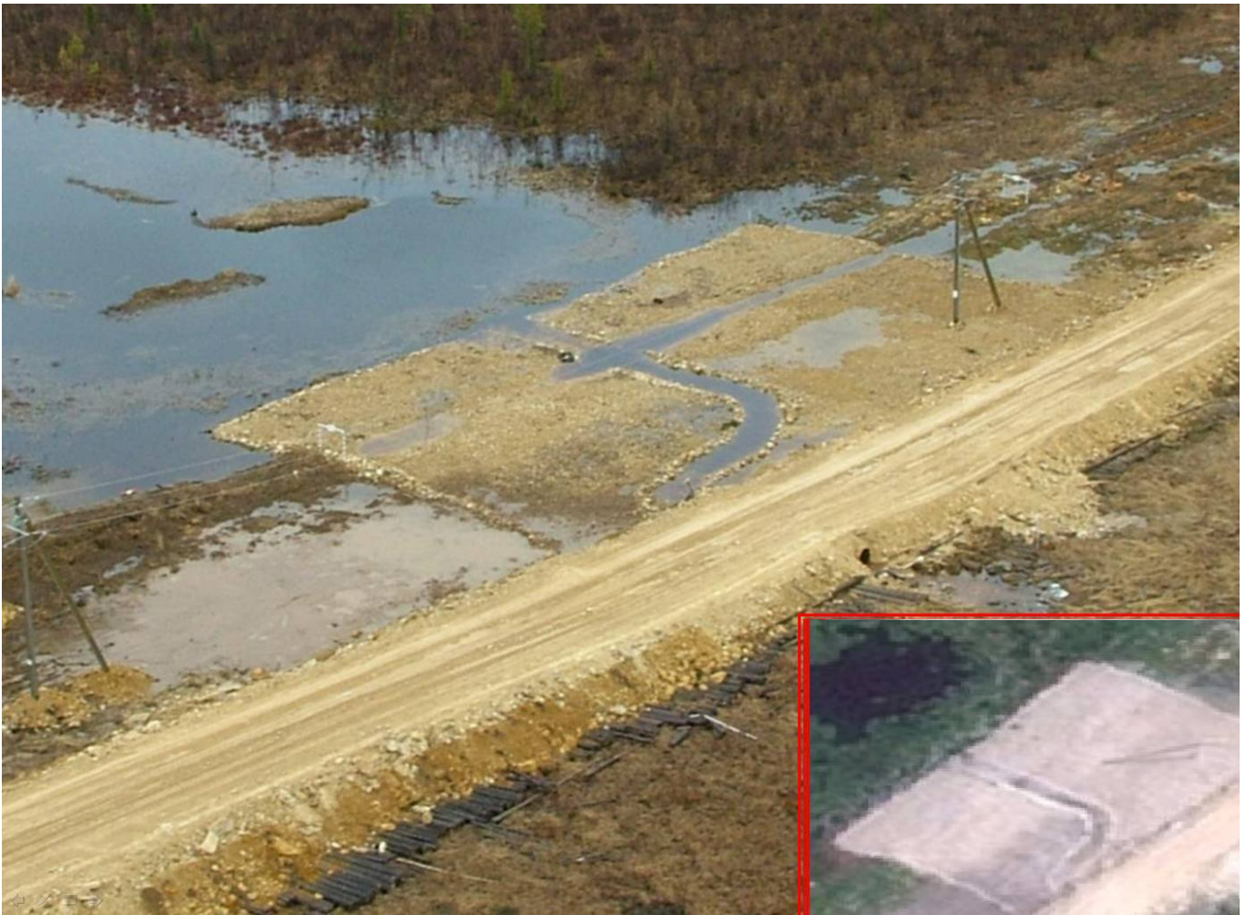
Figure 1. Thermokarst development at the anti-erosion gravel pad. The photo in the bottom right corner shows the same place eight months earlier.
