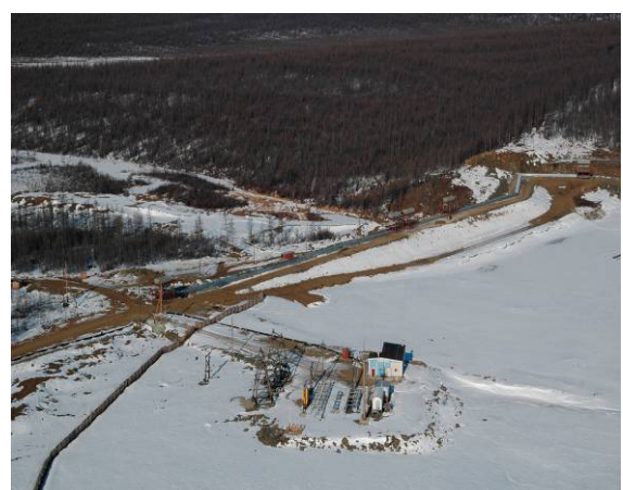
Figure 9. Liendokit River dam. Nyurba mining and processing complex of AIROSA Company.
