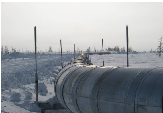
Figure 8. Vankor-Purpe oil pipeline.
