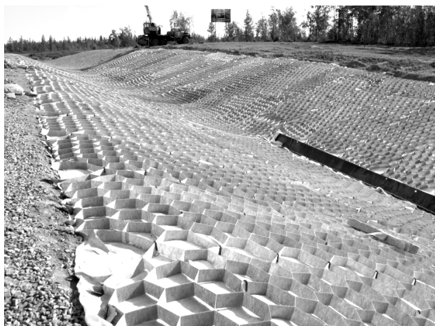
Figure 1. The 2009 construction of erosion- and landslide-control structures using geogrid.
