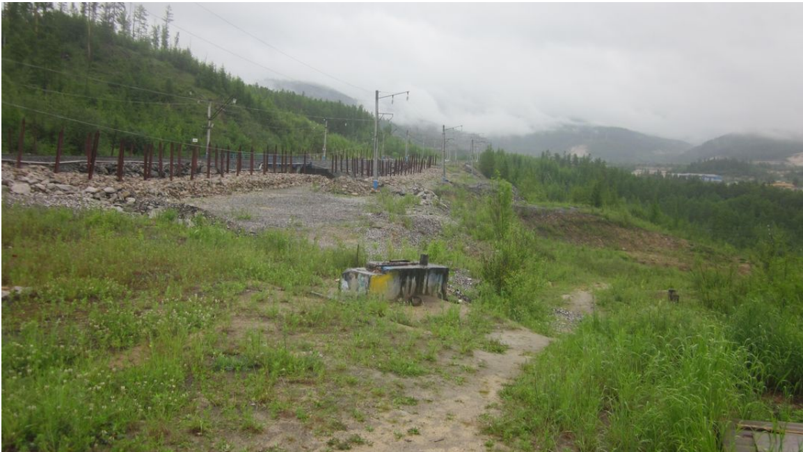
Photo 9. Baikal Amur Mainline (BAM) Railroad at Severomuysk. This original four-track station area now operates on a single line at reduced speed.
