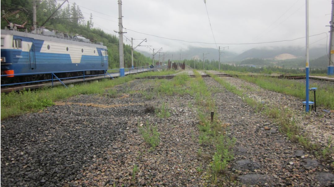
Photo 8. Baikal Amur Mainline (BAM) Railway at Severomuysk. View of a very large continuing major slope instability area that has reduced travel through this segment to one track and maximum speed of 25 km/hr. Application of heat pipes, groundwater interception and recent air convection rock slopes has failed to stabilize this area.
