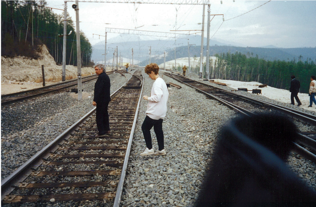
Photo 7. Baikal Amur Mainline (BAM) Railroad at Severomuysk. View of multi-track conditions during a site visit in June, 1992.
